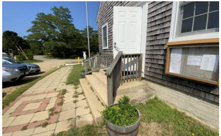
FRONT DOOR: Renovate Exterior Stair, Handrail, and Guardrails
