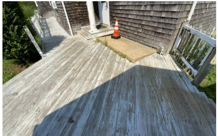
ADA CONNECTIVITY: Renovate Decking to be Flush with Door Thresholds
