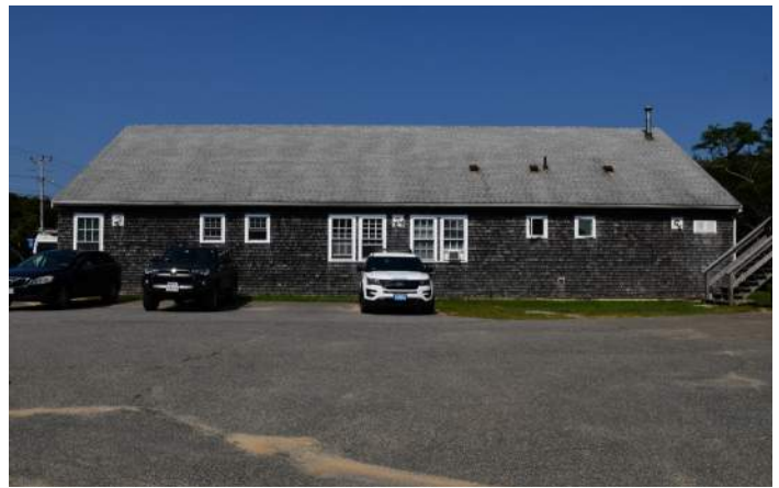
CEDAR SHINGLES BEYOND USEFUL LIFE: Cupping, rot, loose shingles
