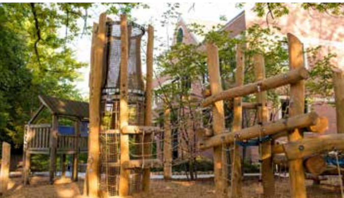
Custom timber play structure made from salvaged black locust posts at Upper Canada College in Toronto. Source: EarthScape.
